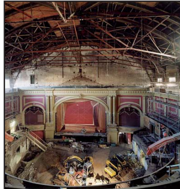
Auditorium during renovation, photo Frank Greiner
