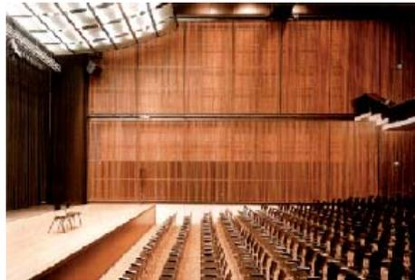
Possible change of acoustics by fabric curtain running behind an acoustically transparent wooden side wall cladding
